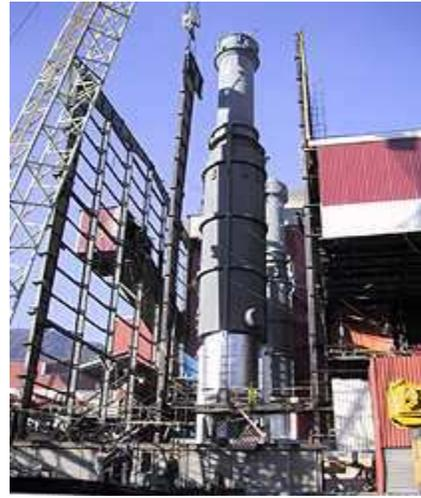
**Figure 4 - (a) Metallic Radiation Recuperator Design (Source: PG & E), (b) Radiation Recuperator Installed at Glass Melter (Source: ALSTOM)**
